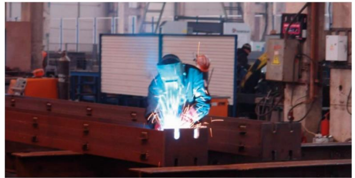
ASSEMBLY AND WELDING
